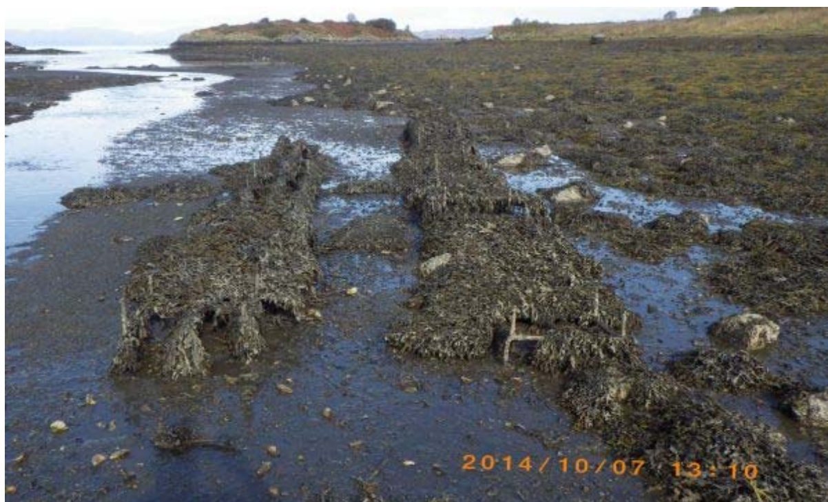
Figure 13. Disused former Ardencaple-Cadzow trestles, Camuslaich Bay. Waypoint 44.
