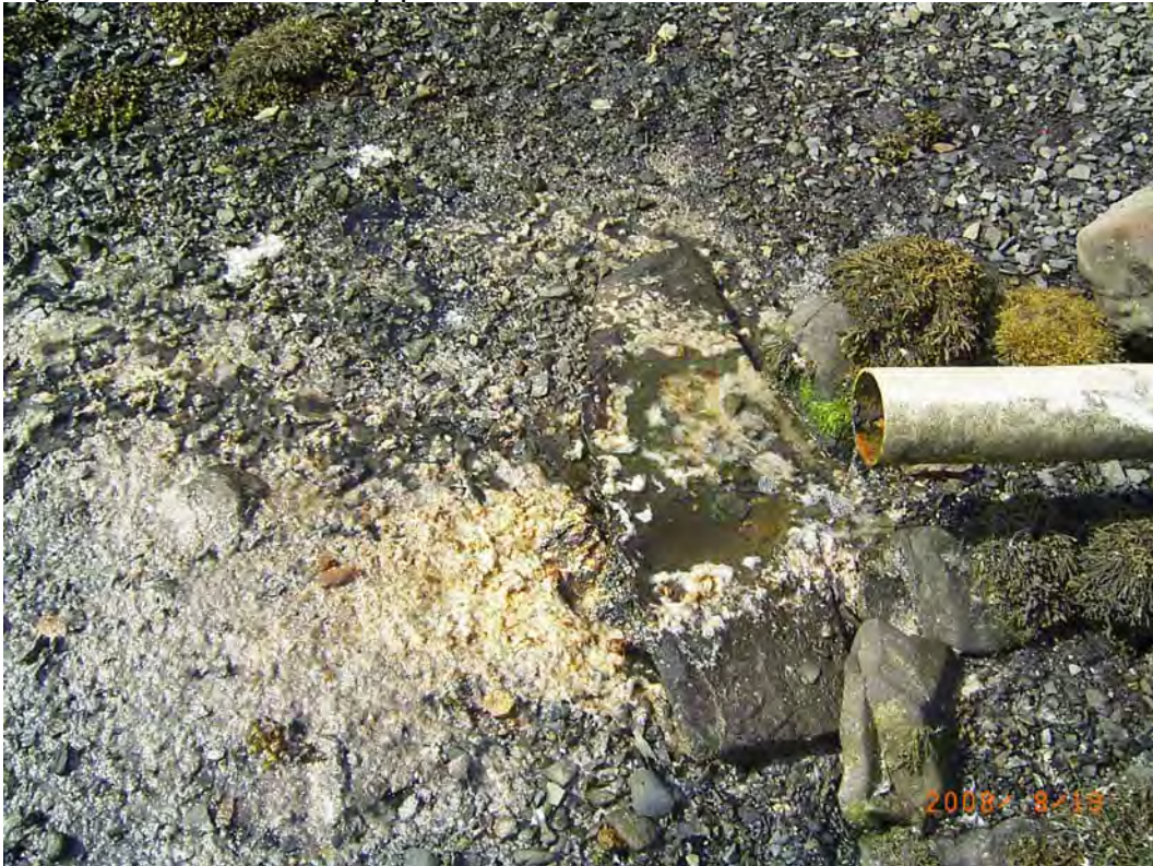
Figure 5 Private sewer pipe at Clachan Seil
