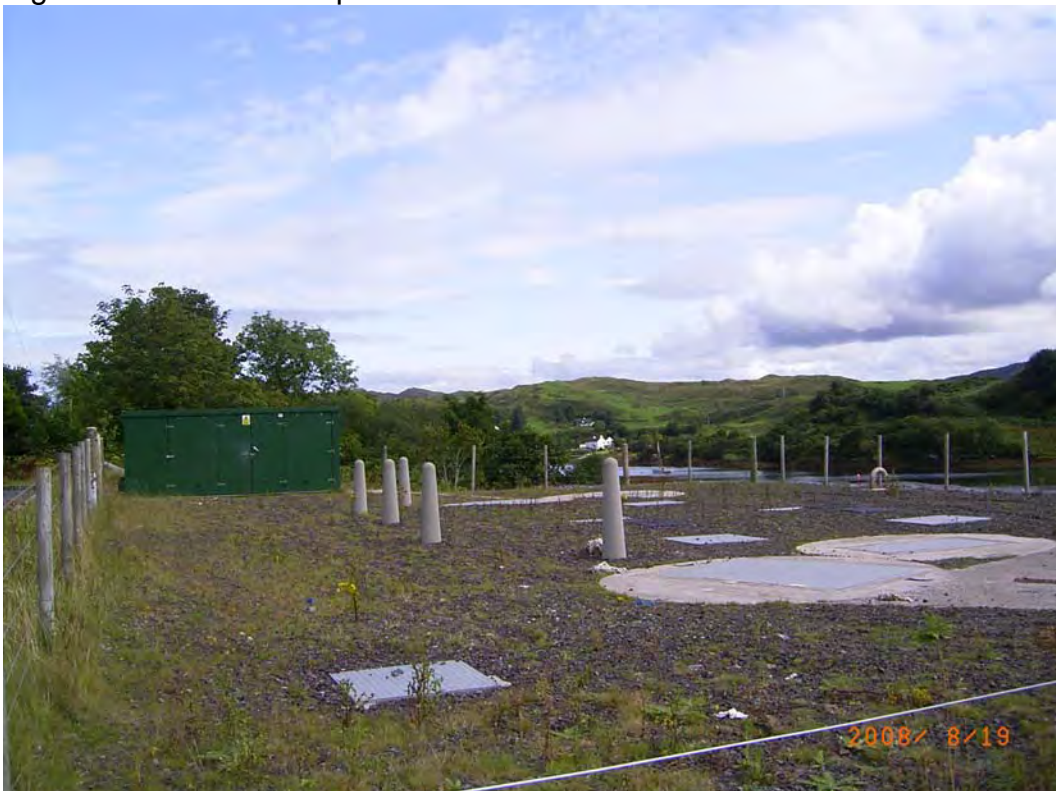
Figure 6 Communal septic tank at Clachan Seil
