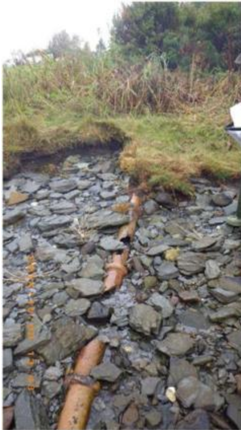
Figure 13. Broken ceramic pipe with flow. Site of unplanned freshwater sample SSFW8. Waypoint 48.
