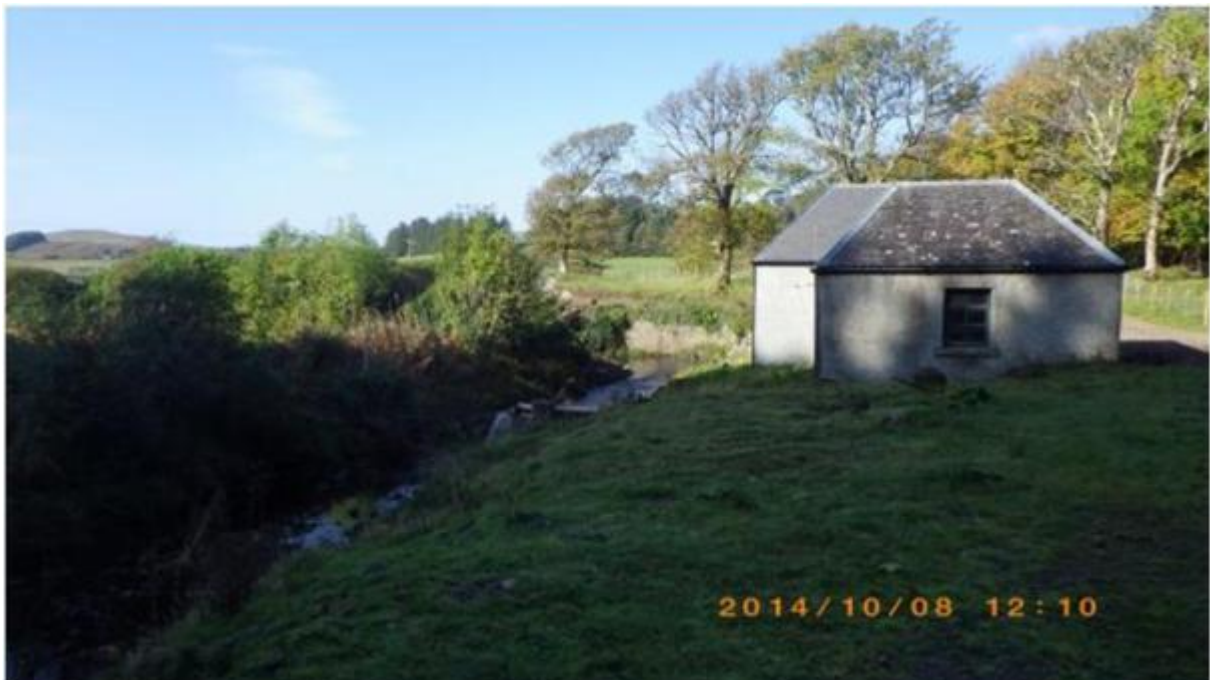
Figure 17. Housing for old (small) and new (larger) small scale hydroelectric plant at Ardmaddy Bay on the Eas nan Ceardach watercourse Waypoint 88. Site of planned freshwater sample SSFW10, Waypoint 89, is three metres downstream of the second (larger) building.
