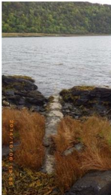
Figure 13. Broken ceramic pipe with flow. Site of unplanned freshwater sample SSFW8. Waypoint 48.
