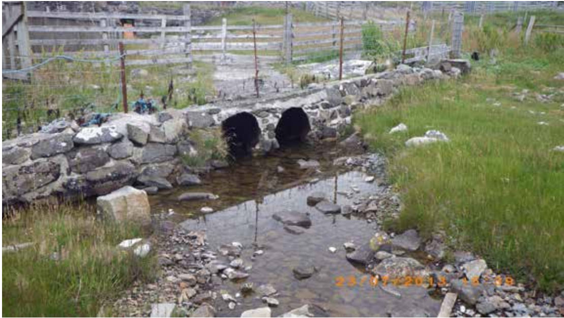
Figure 5. Two pipes running under road and under sheep fold next to road. Associated with waypoints 13 and 14. Planned freshwater sample LSFW4.
