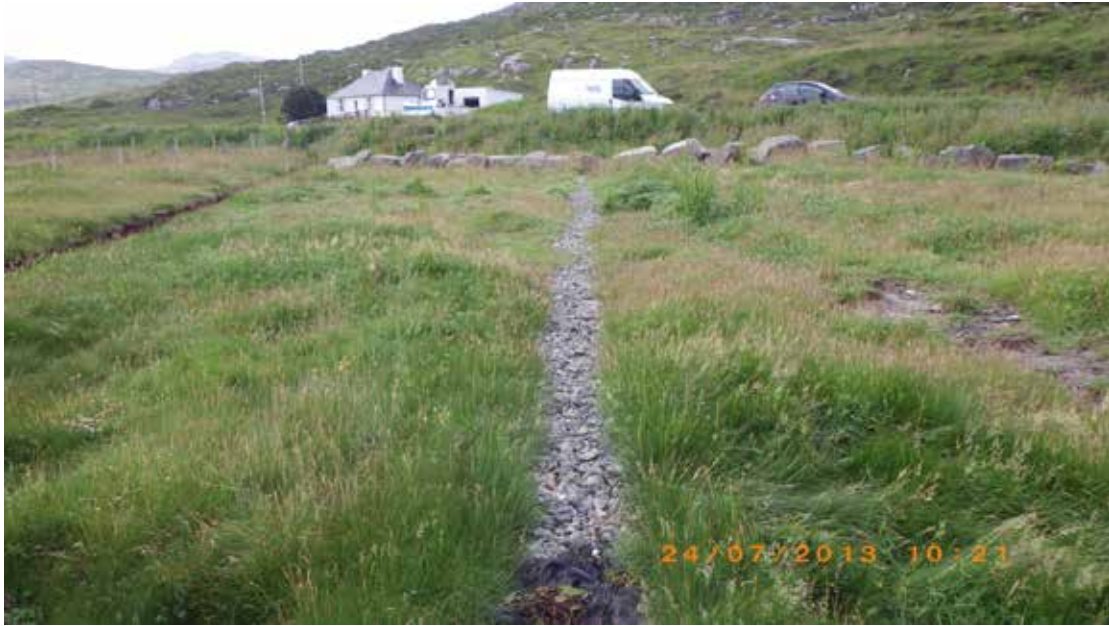
Figure 7. Public discharge onto shore, covered over with stones until it reaches the beach. Associated with waypoint 20 and 21. Planned seawater sample LSSW2.
