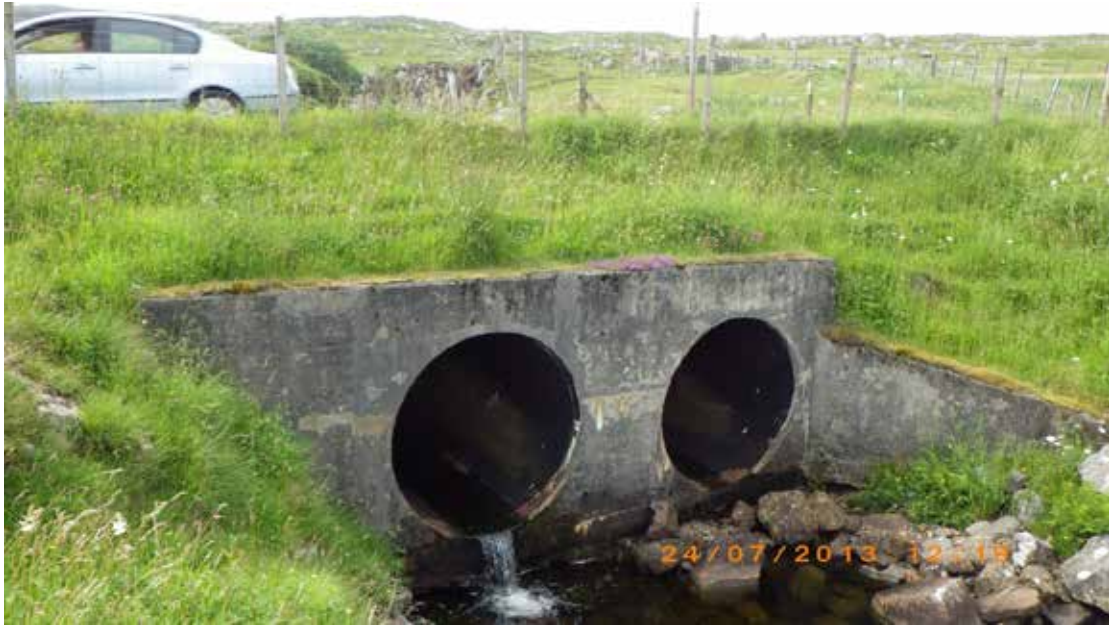
Figure 12. Two large pipes of 1.5 m width directing watercourse under road onto shore. Associated with waypoints 30 and 31. Planned freshwater sample LSF10.
