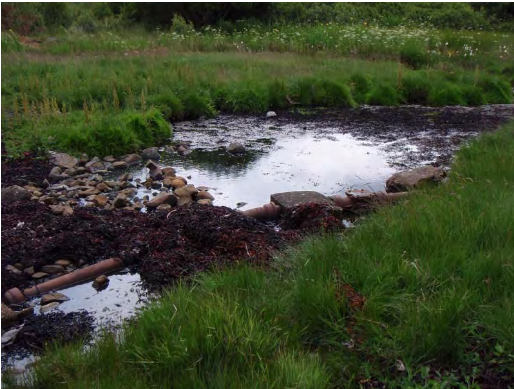
Figure 12. Iron septic pipe, not discharging
