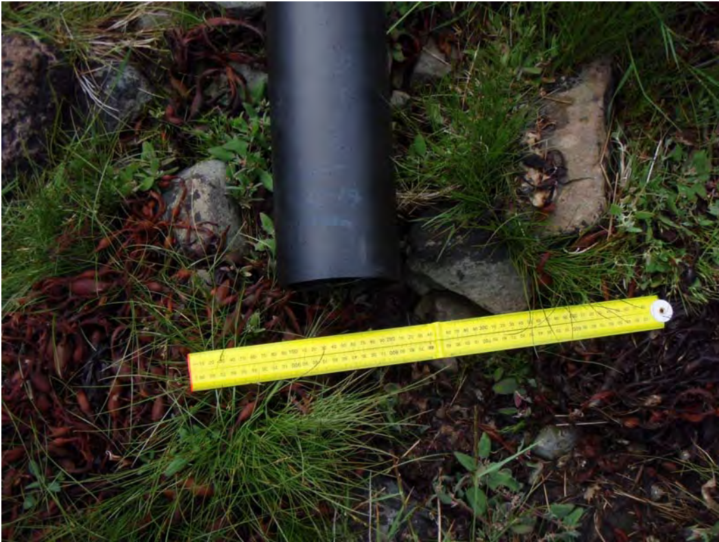
Figure 11. Black discharge pipe
