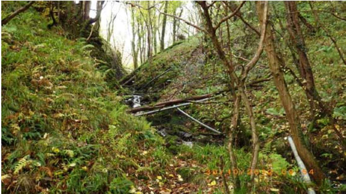
Figure 7. River running into bay at Port na Coite. Pipes scattered but not attached or flowing.
