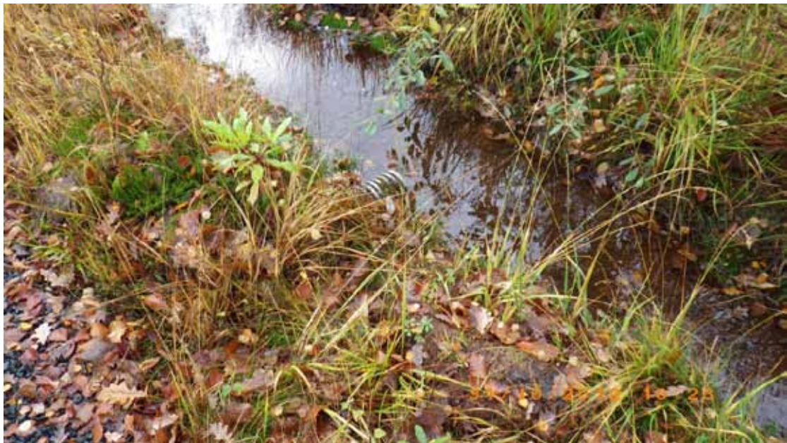
Figure 16. Surface drainage with pipe.
