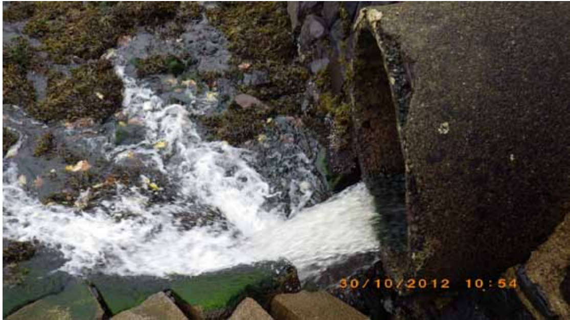
Figure 9. Outflow from pipe, sample TOW4 taken here.
