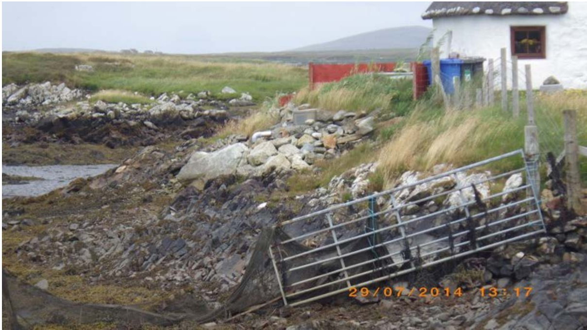
Fig. 16 Septic tank from holiday house with outfall pipe ending in air above shore. No flow observed. Photograph taken from waypoint 57.
