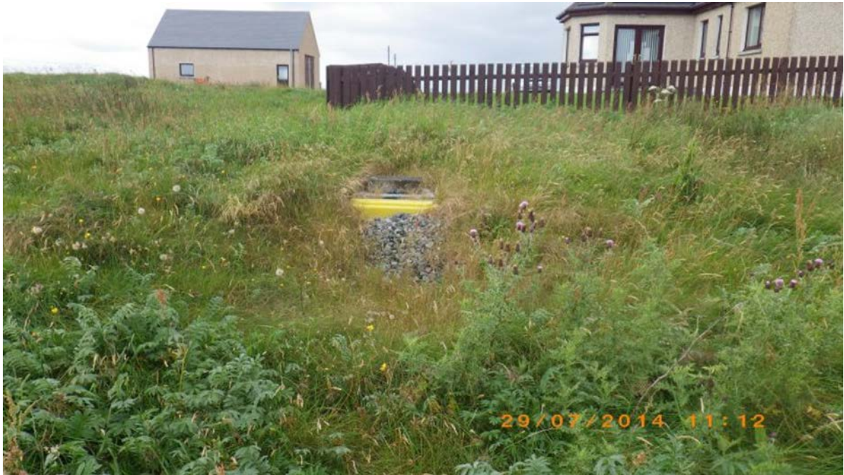
Fig. 12 Septic tank and apparent soakaway in garden ground of new house. Waypoint 41.
