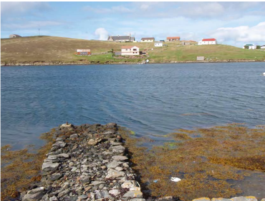
Figure 17. Jetty, photo looking west from waypoint 38.
