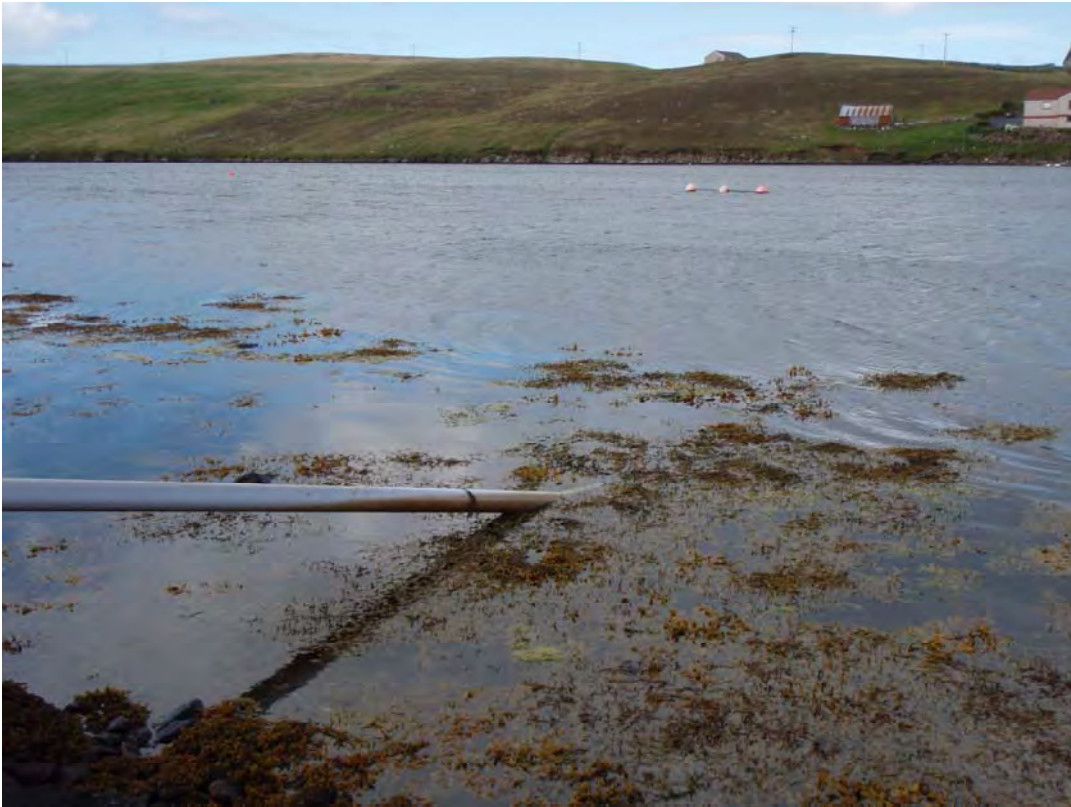
Figure 16. Septic pipe from house, waypoint 37.
