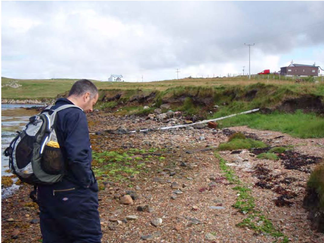
Figure 20. Discharge pipe from home on shore near oyster raft.
