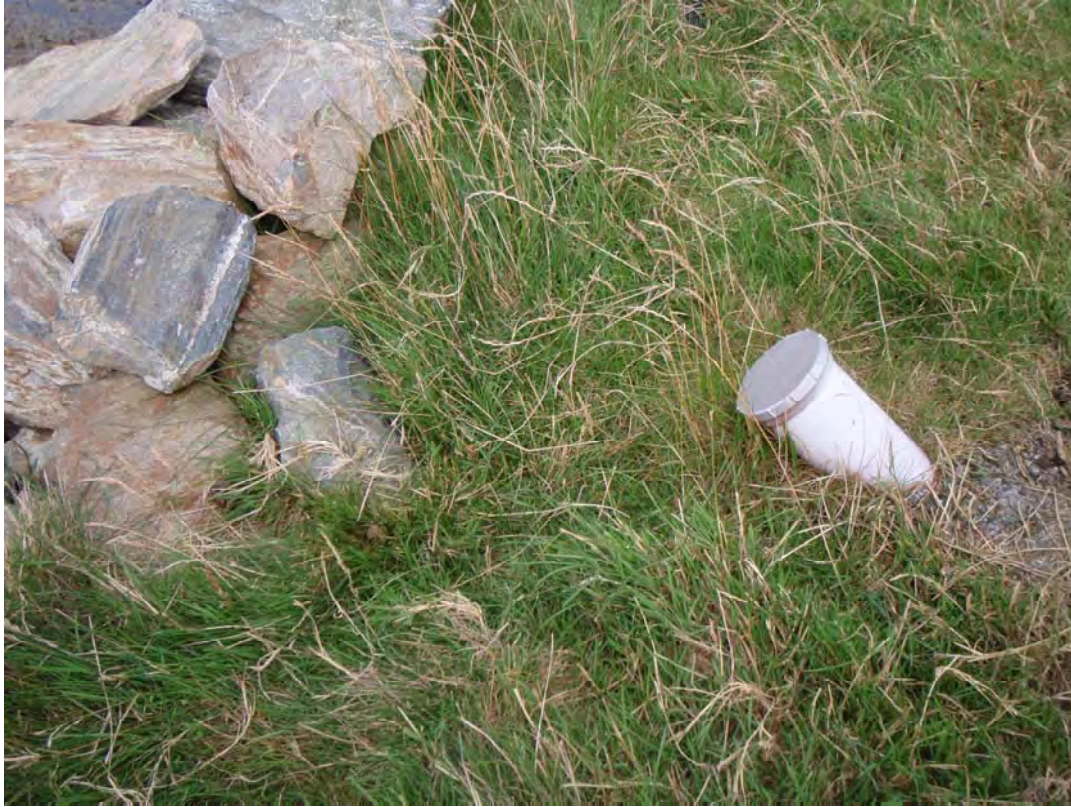
Figure 18. Septic tank inspection pipe.
