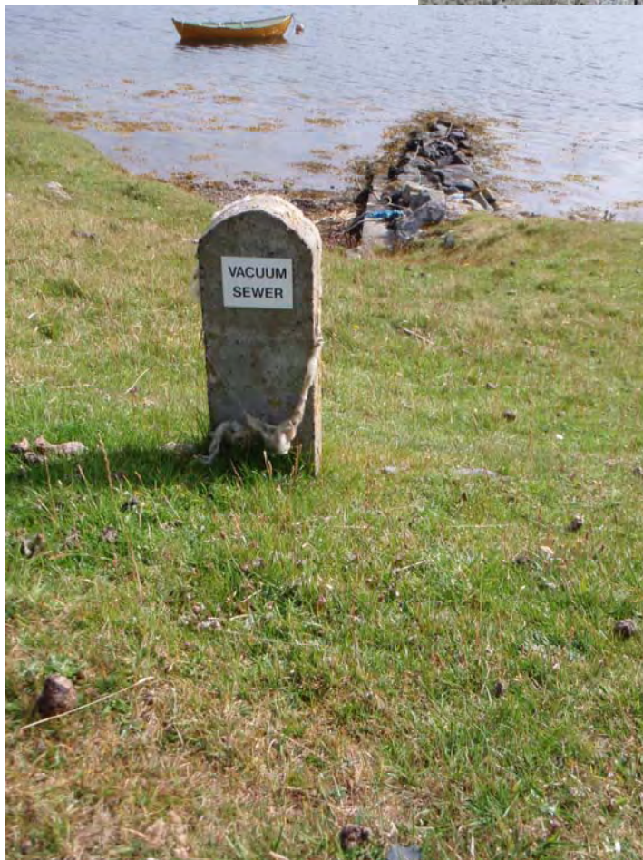
Figure 6. Septic tank, Toogs
