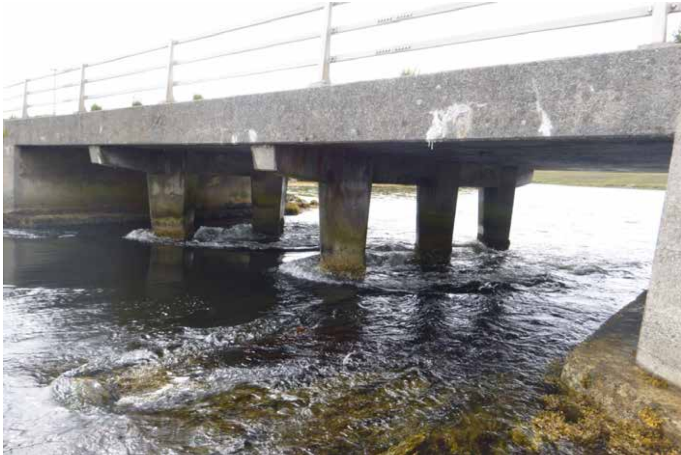
Figure 14 – Water flowing under Strom Bridge from Strom Loch to Stromness Voe.
