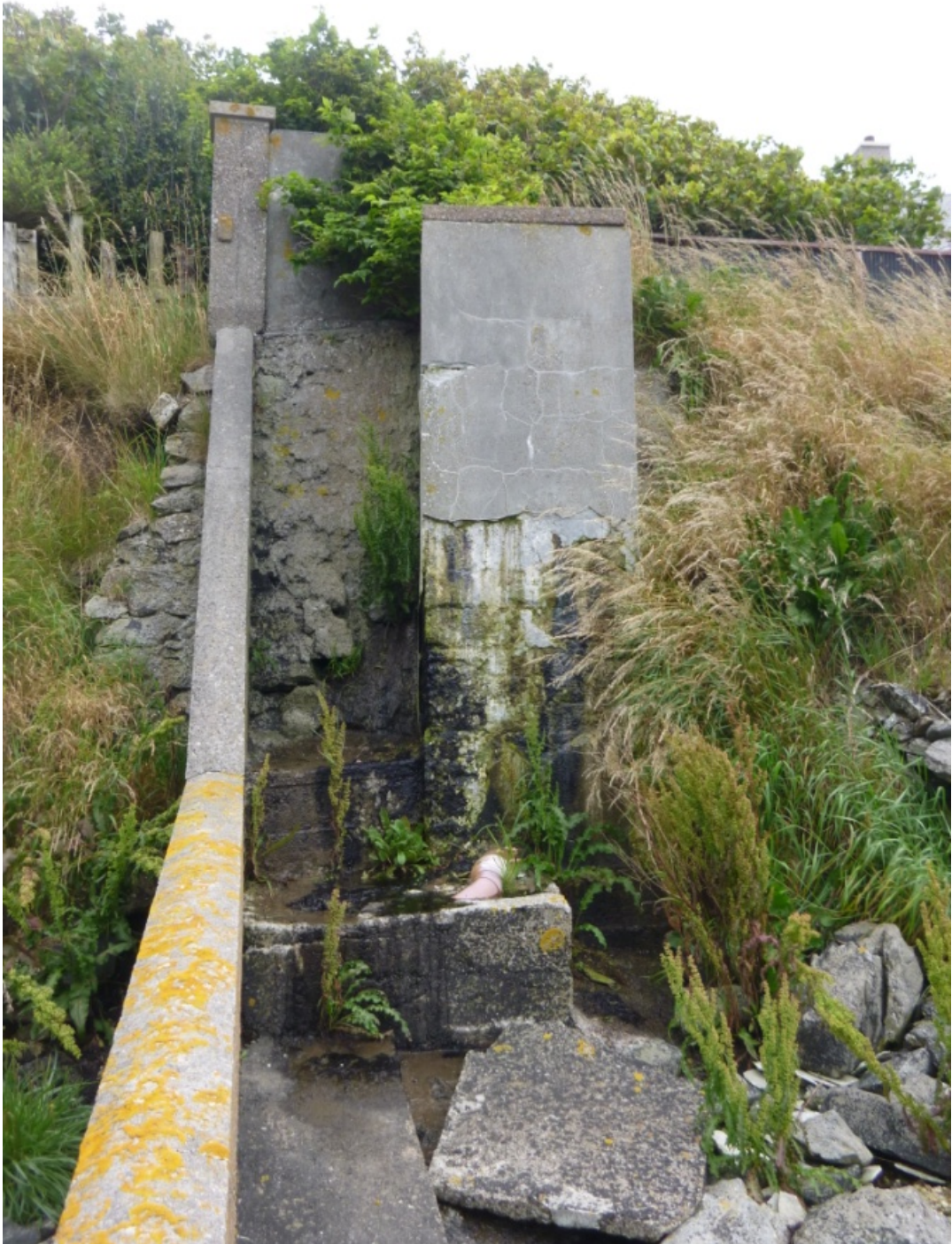
Figure 7 – Septic tank located north of the Strom Bridge.
