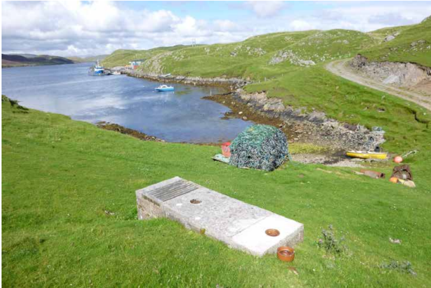
Figure 11 – Septic tank associated with a holiday home at Pund.
