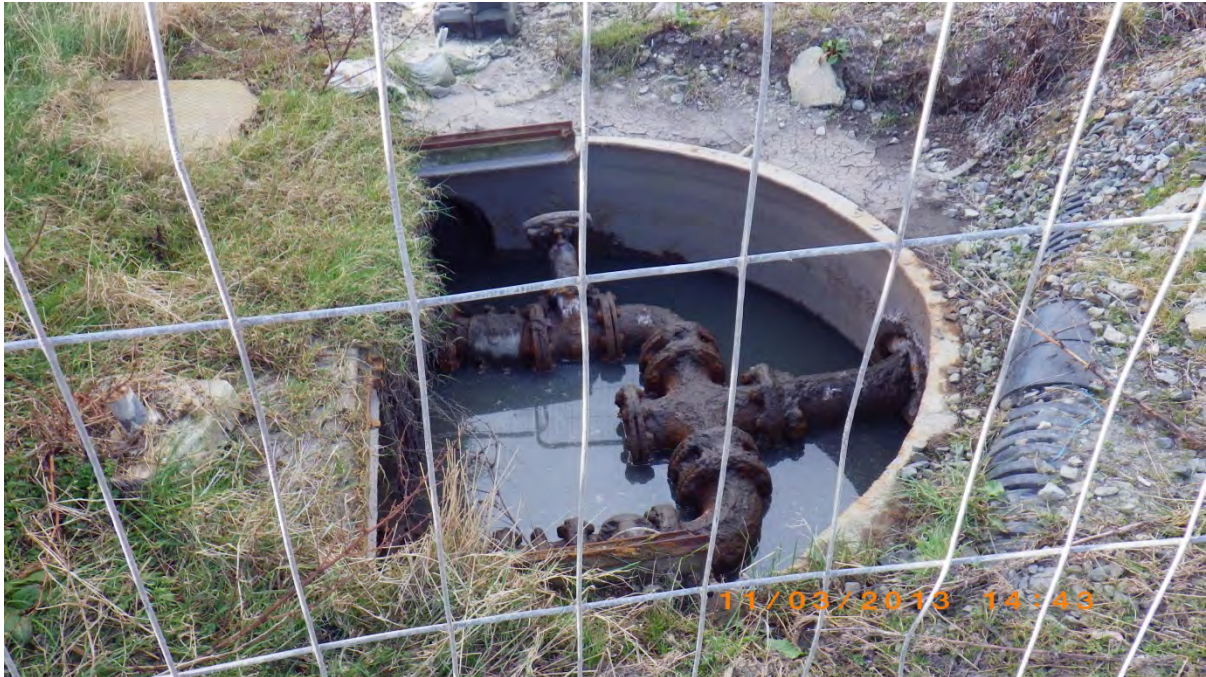
Figure 11. Waypoint 26. Scottish Water Station, Sand Street Pumping Station.
