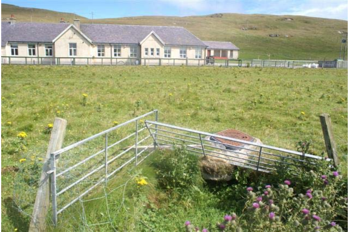
Figure 8. Drain opposite school
