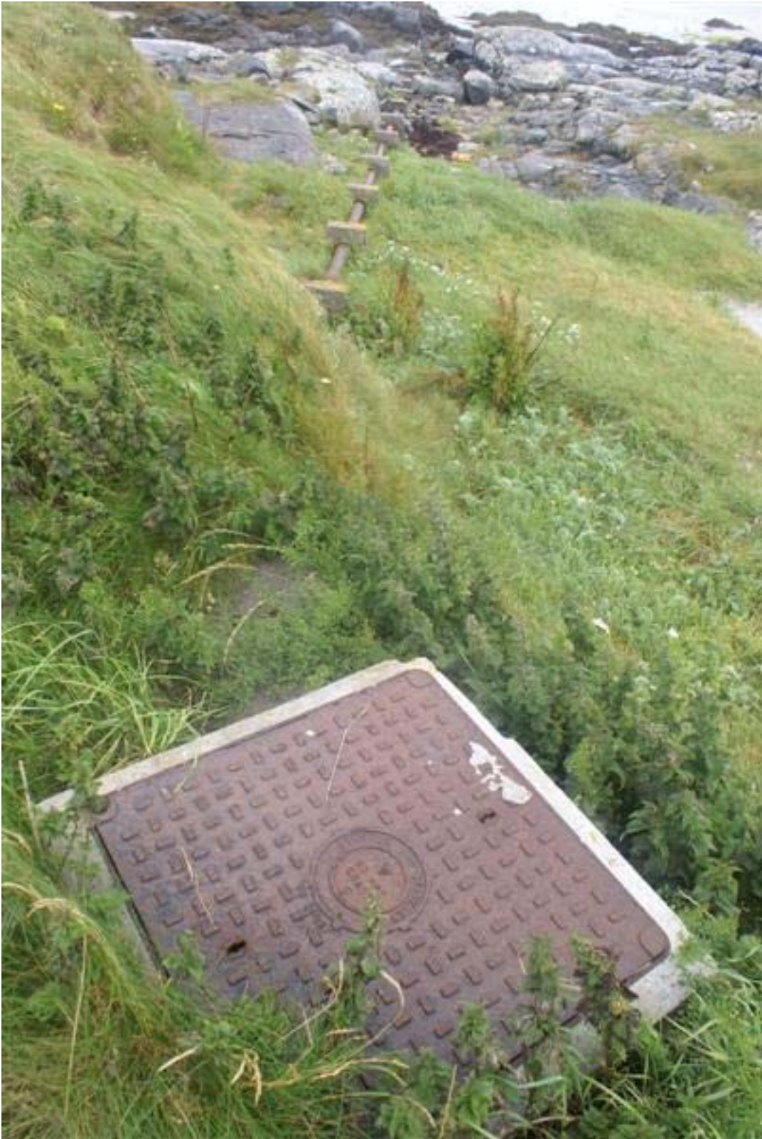
Figure 18. Inspection cover of septic tank and outfall pipe
