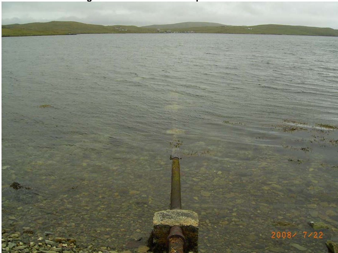
Figure 7 Communal septic tank outfall
