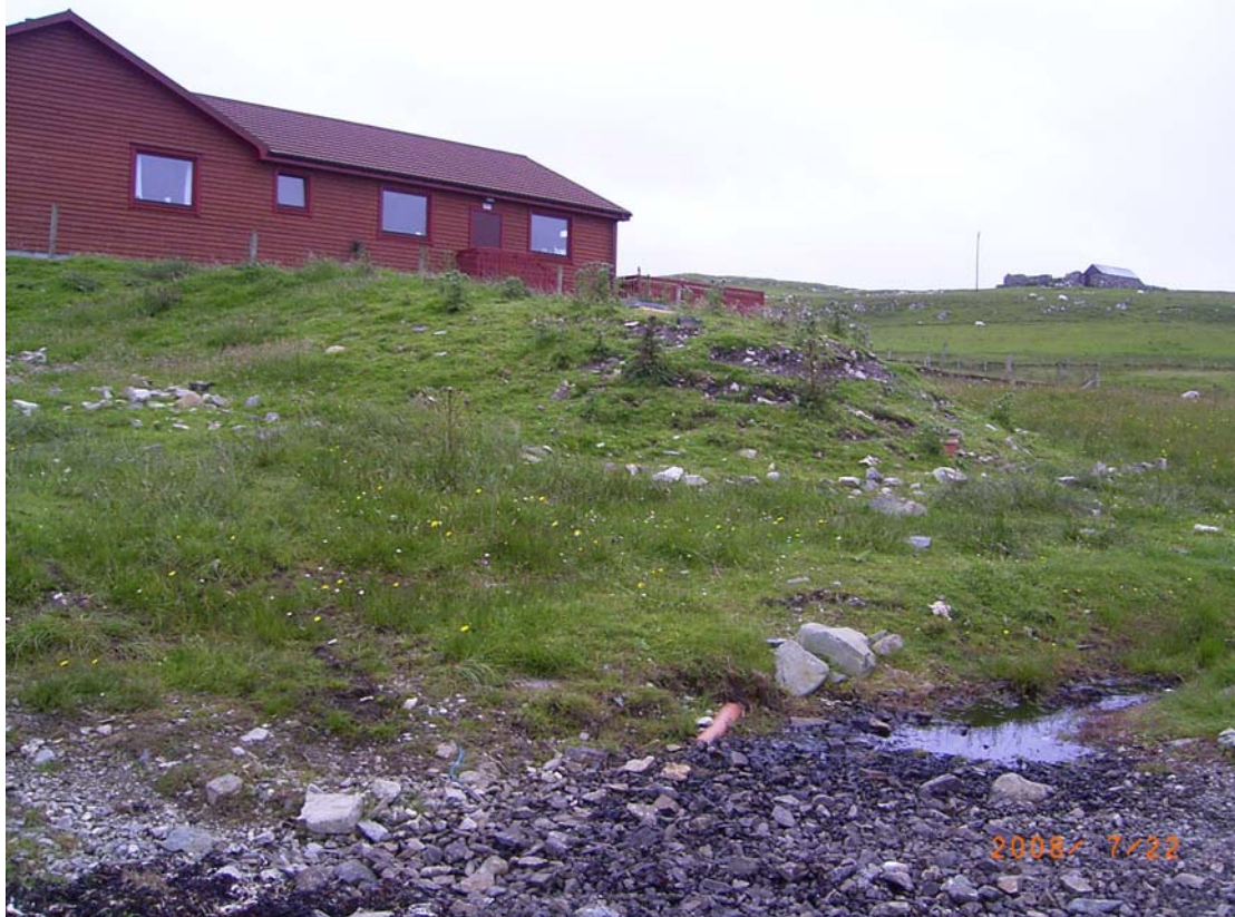
Figure 14 Private septic tank
