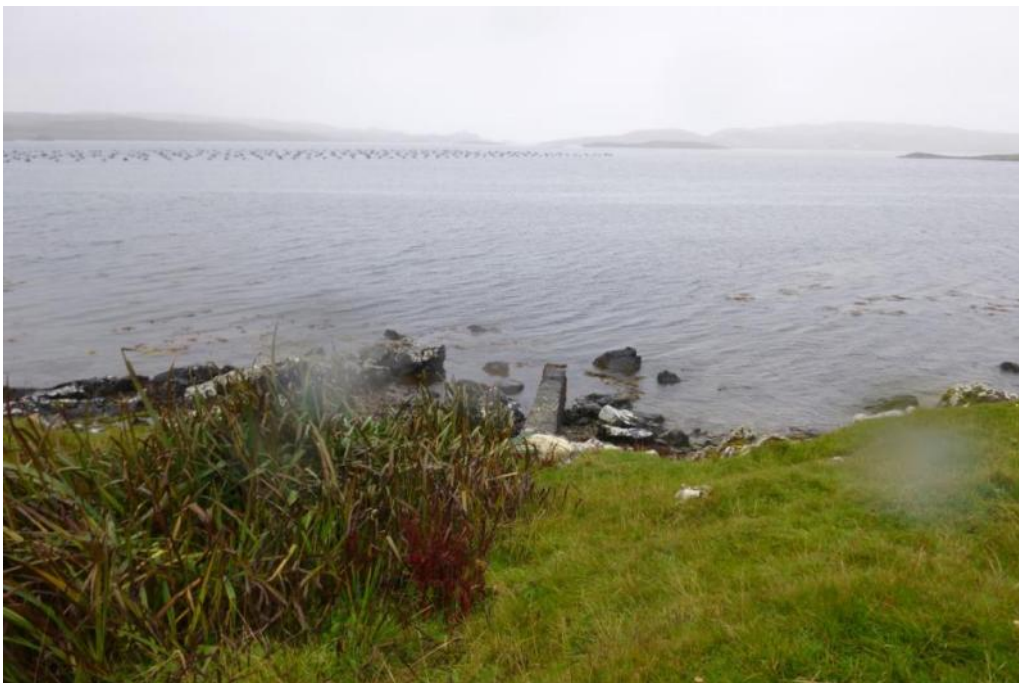
Figure 17 – Concrete ducting running into sea below Stapness.
