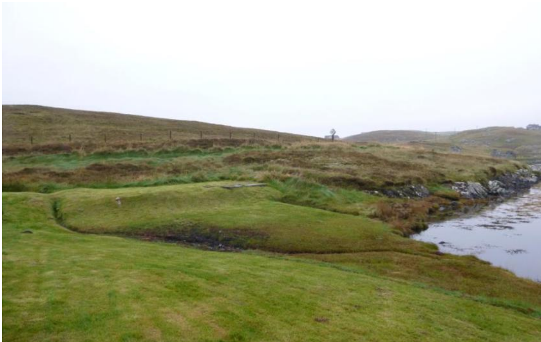
Figure 13 – A septic tank including channel leading to sea at the head of Lera Voe.
