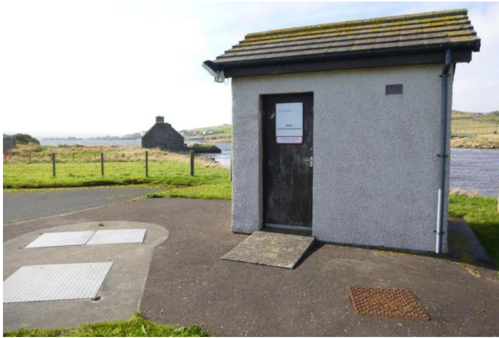
Figure 26 – Walls East Pumping Station.
