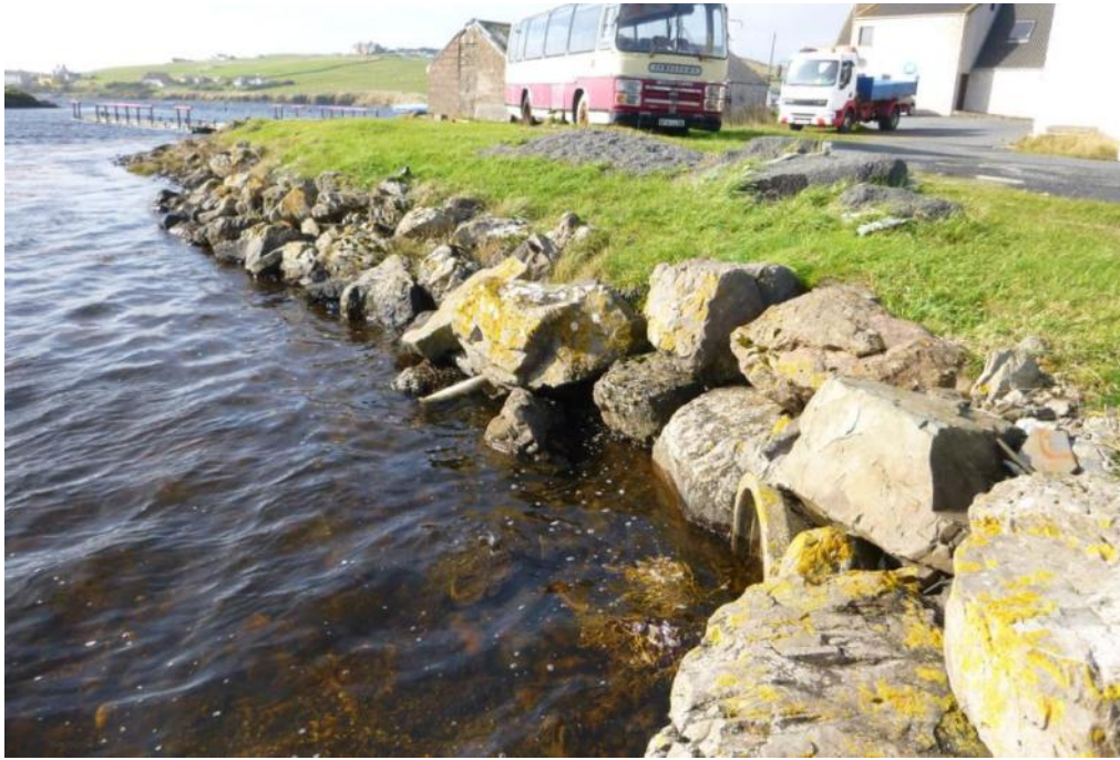
Figure 28 – A land drain and small pipe underwater opposite Walls marina.
