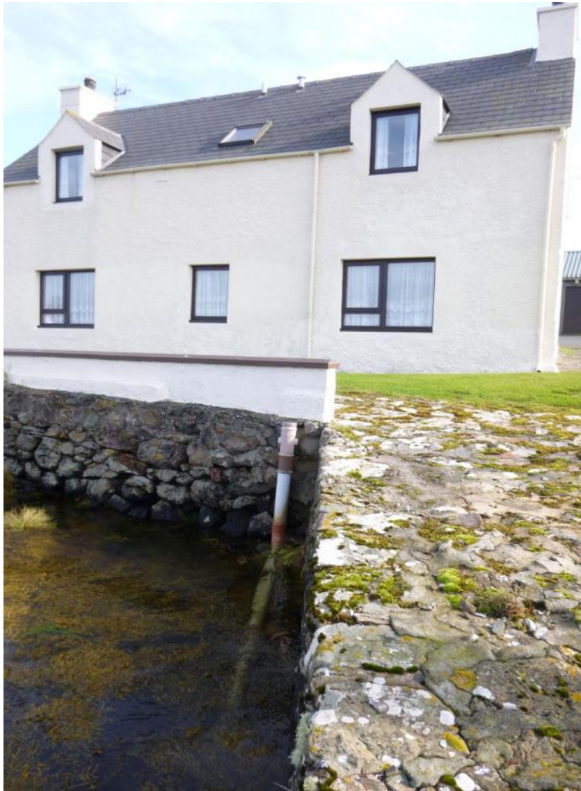
Figure 27 – A plastic pipe receding underwater below house at head of voe in Walls.
