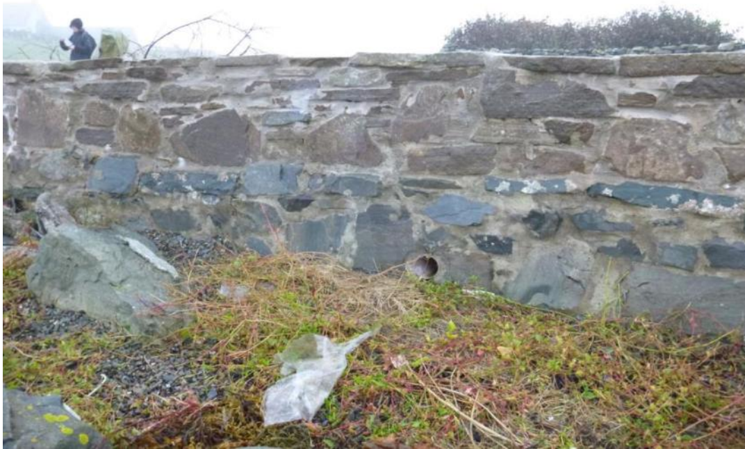
Figure 24 – Outflow pipe to beach at Vadlure, believed to be in use for kitchen wastewater only.
