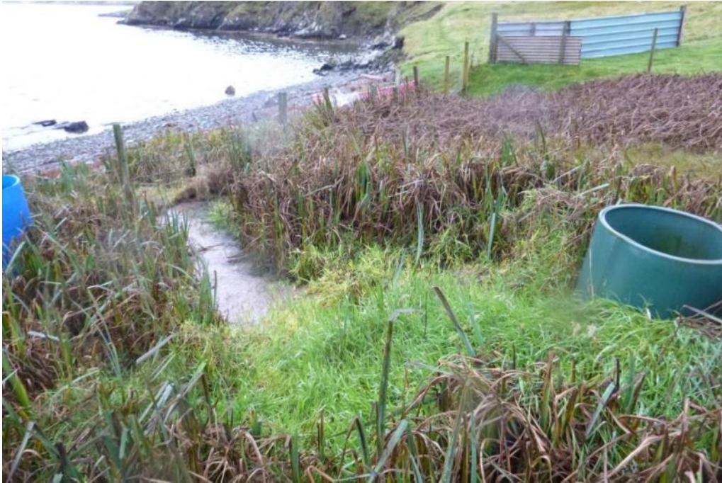
Figure 14 – Overflowing septic tank at Crookataing, a seawater sample was collected here.
