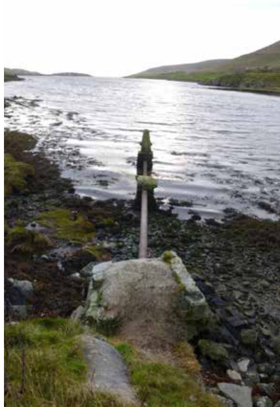
Figure 12 – Discharge pipe associated with the Swedish Houses community septic tank.
