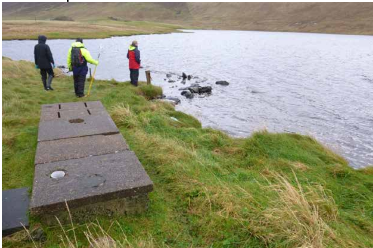
Figure 9 – Septic tank servicing the Shetland Jewellery workshop and visitors centre adjacent to the Loch of Hellister.
