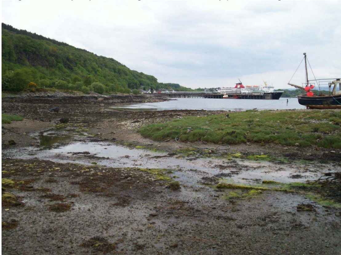
Figure 19. Bay adjacent Craignure WWTW, ferry pier in background
