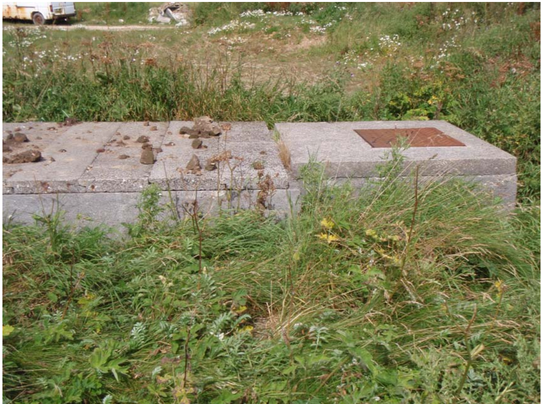
Figure 9 Septic tank
