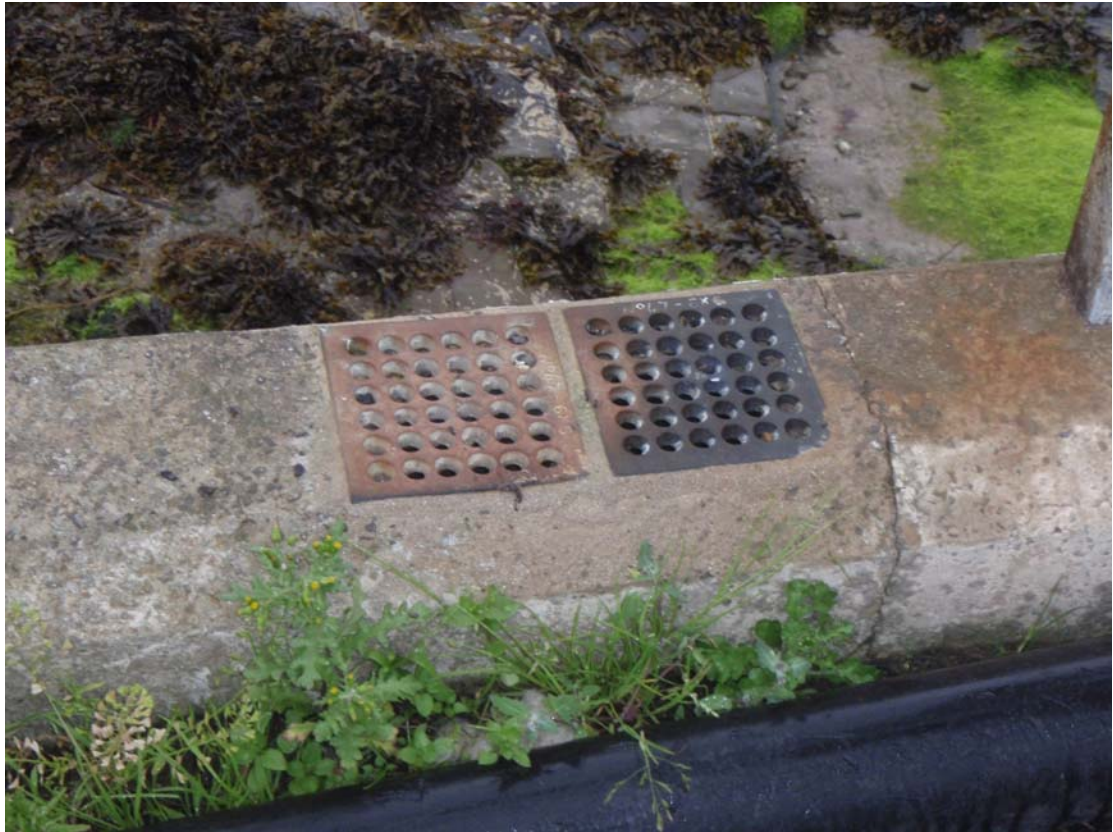
Figure 8 Vent on pier wall
