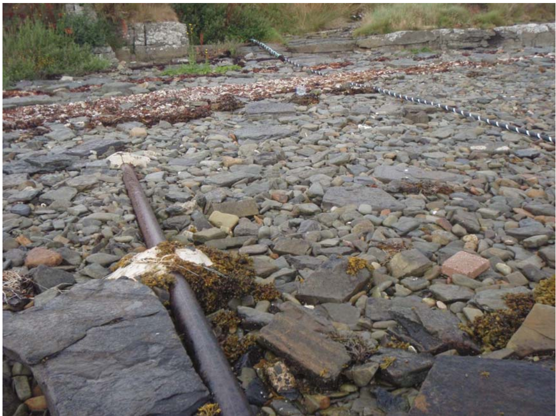
Figure 7 Iron sewage pipe to shore
