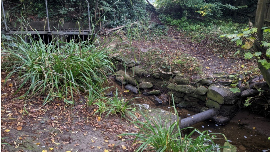
Figure 8. The Rivacre Brook is diverted under the A41 in a wooded area
