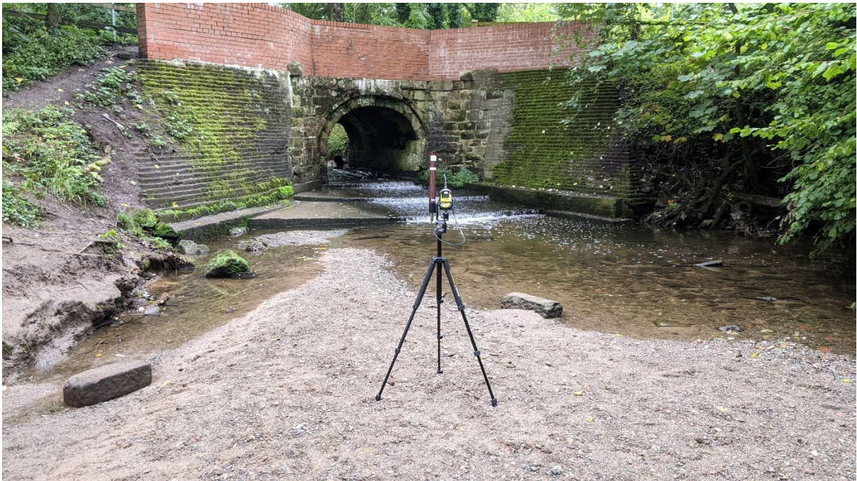
Figure 13. The brook passing under a road in the Rivacre Valley Country Park
