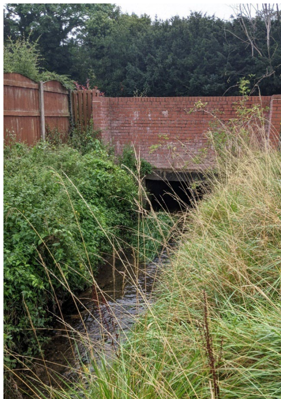
Figure 9. The brook emerges from under the A41 next to Ascot Drive
