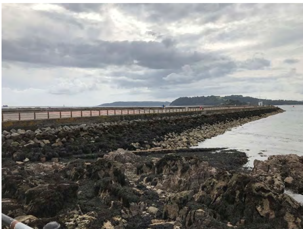
Figure 8. Mount Batten Breakwater
