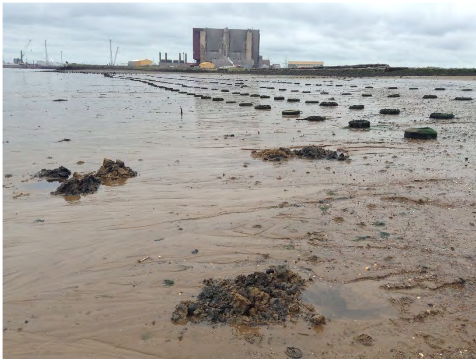
Figure 7. East of the power station jetty
