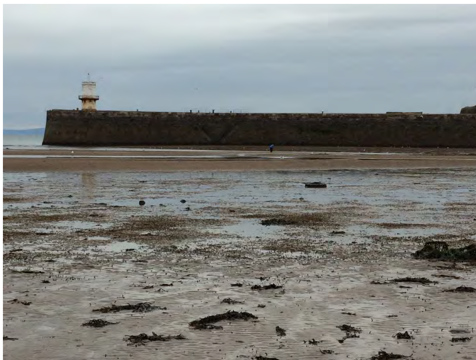
Figure 4. Whitehaven Outer Harbour
