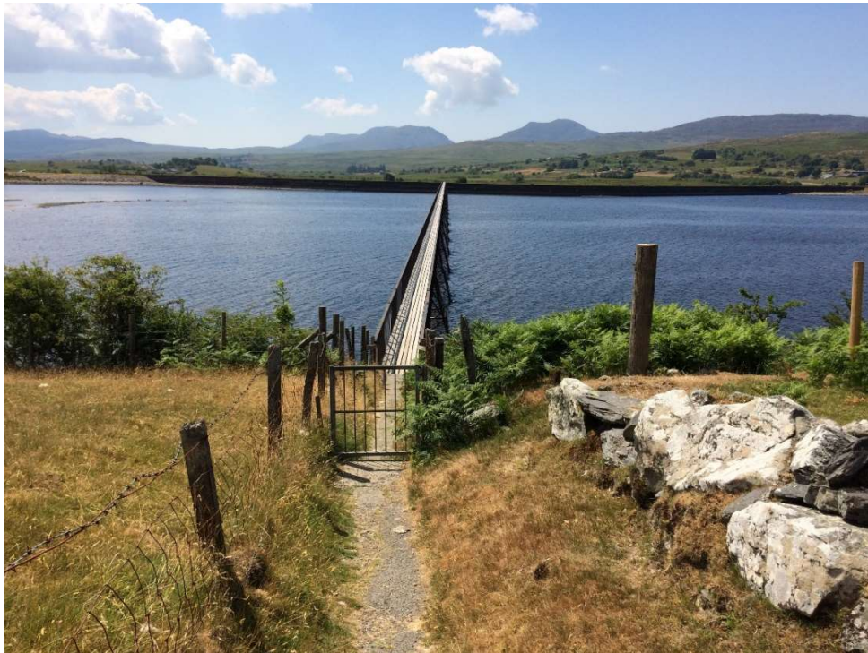
Figure 7. The footbridge from Trawsfynydd Village across the lake
