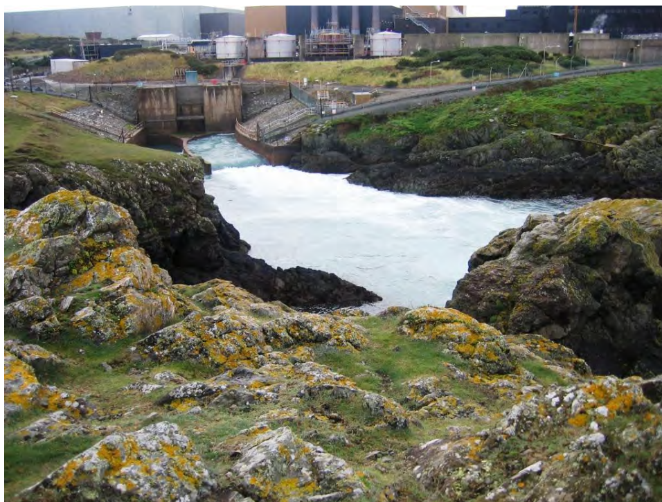
Figure 5. The outfall at Porth Wnal
