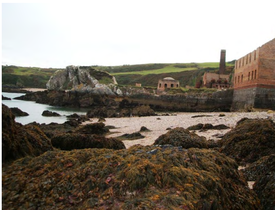
Figure 7. The brickworks at Porth Wen
